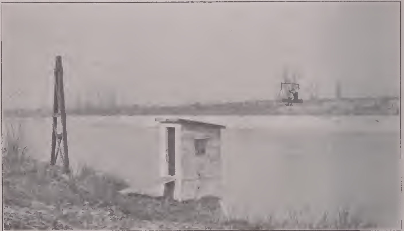
B. MEASURING EQUIPMENT AND RECORDER INSTALLATION, PUYALLUP RIVER AT PUYALLUP.
